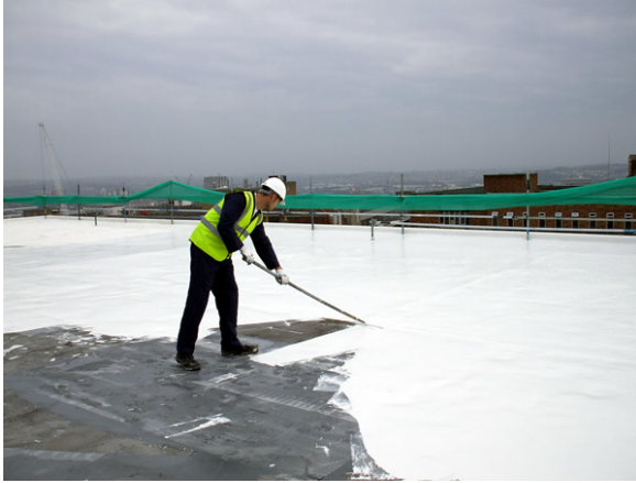
Figure 3: Applying reflective coating on the roof
