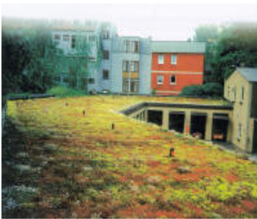
Figure 5: Extensive green roof
