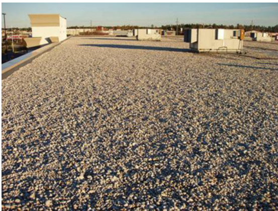
Figure 4: Gravel ballasted flat roof
