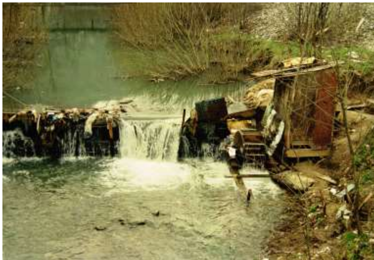
Photograph 40 Small power station (Photo courtesy of Serge Jenssen, January - June 1994, Potočari)
