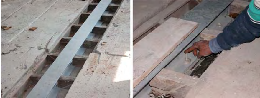
Figure 4.5, detail of insertion of fiberglass pegs
