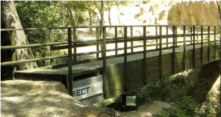
Pedestrian Cycle Footbridge, Pitigliano, Grosseto, Italy, 2004
