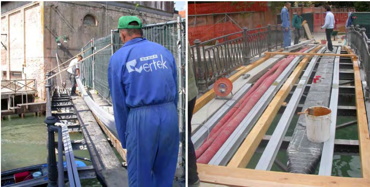
Figure 4.18, Transport and installation phase
