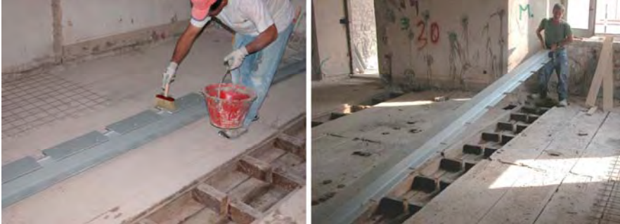
Figure 4.4, Executive and installation phases
