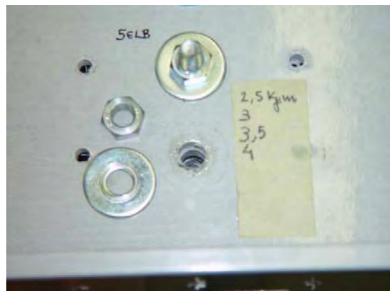
Figure 5.52. View after application of 40 Nm (equal to 25000 N) on bolt
