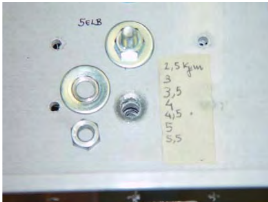
Figure 5.55. View after application of 55 Nm (equal to 34375 N) on bolt
