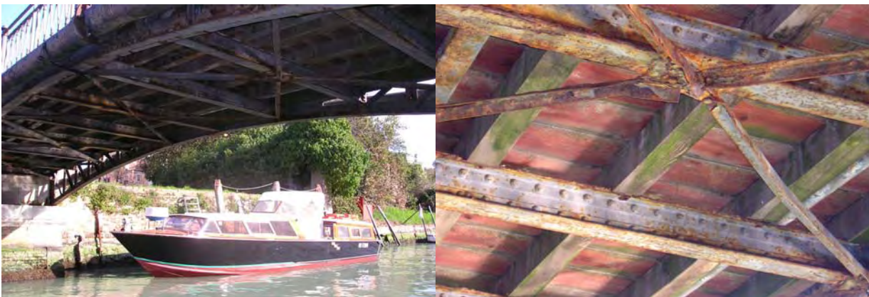
Figure 4.10, Global and local deterioration
