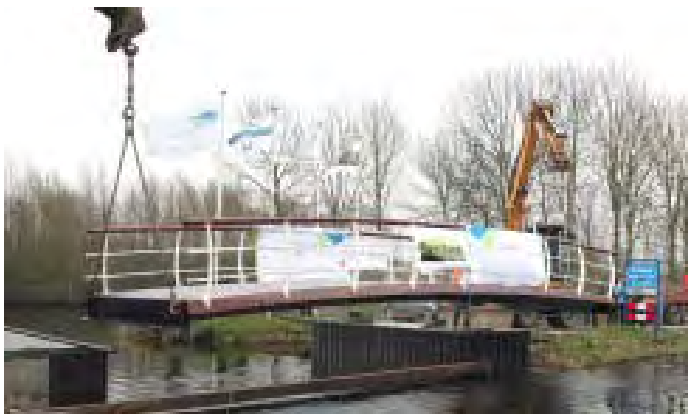
Dronten Bridge, Dronten, The Netherlands, 2007
