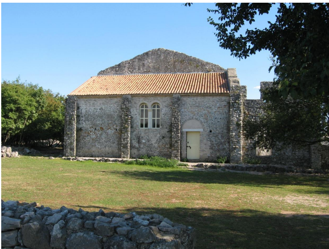
Figure 2. A view of the remains of Mirine complex
