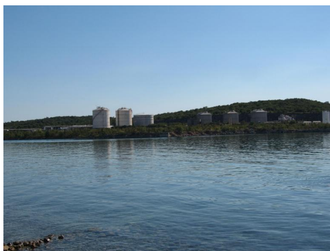
Figure 7. A view from the site towards petrochemical industry terminal
