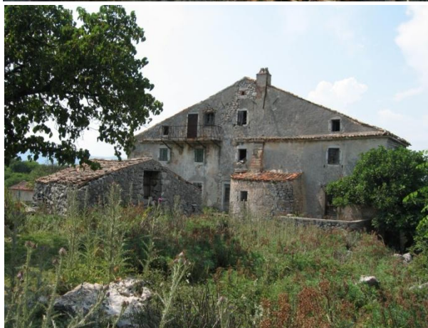
Figure 12. Abandoned residential and production complex in Važmineš
