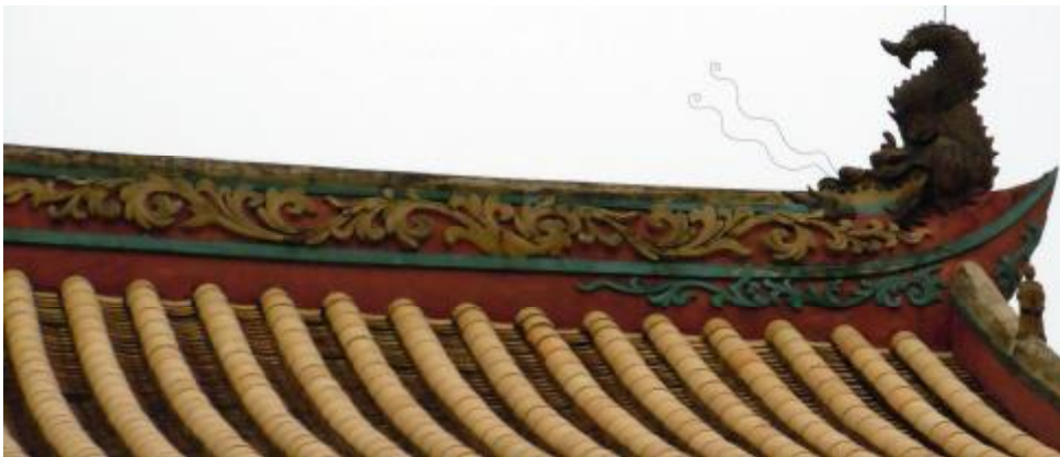
Figure 77. The plasterwork of scroll design and Aoyu of the main ridge of the roof in Mahavira Hall
