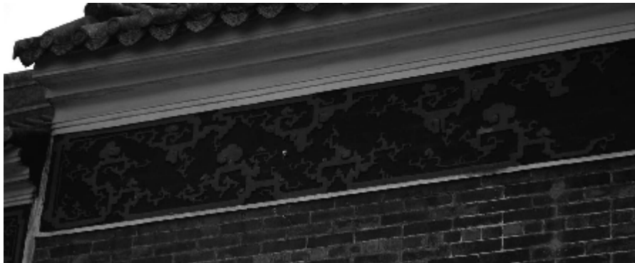
Figure 54. Plastering decoration of Bogu on the back Shawan frieze wall in Chen's Clan temple (1894).
