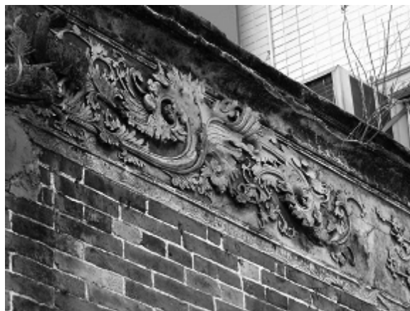
Figure 52. One plastering decoration on the frieze of front wall in Big House of the Tsangs [21] in the city of Hongkong (1867).
