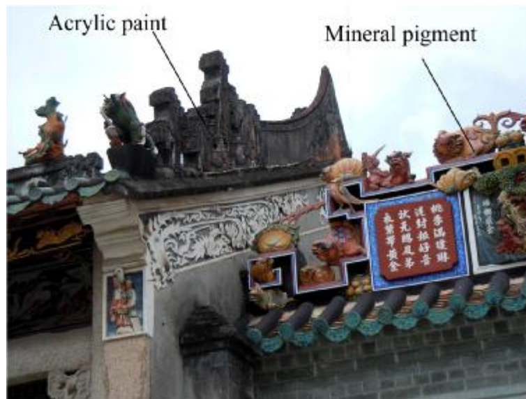
Figure 15. Comparison that used in several acrylic paint and mineral pigment to decorated the plasterwork on the ridge of the roof in Shenzhen Houwang Temple in the same period, and the plasterer Shao Yushan explained that mineral pigment is more perfect and more durable for Guangdong plasterwork, and is also more resistant the wind erosion.
