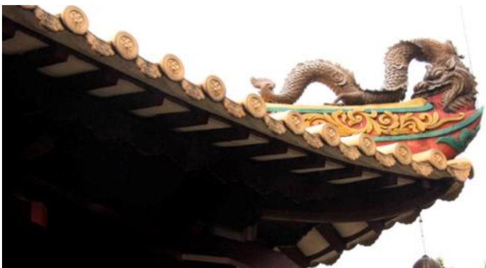
Figure 78. The decoration of dragon of the first eaves angle of hip roof in Mahavira Hall.
