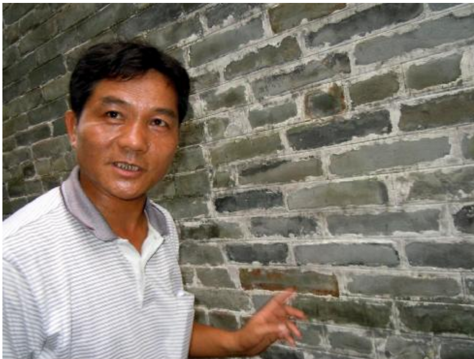
Figure 14. The experienced plasterer Shao Chengcun points to the repaired wall with modern cement mortar to present that it's not still solid enough although it has already repaired several years, and he thinks that the traditional lime mortar is more better and more solid.
