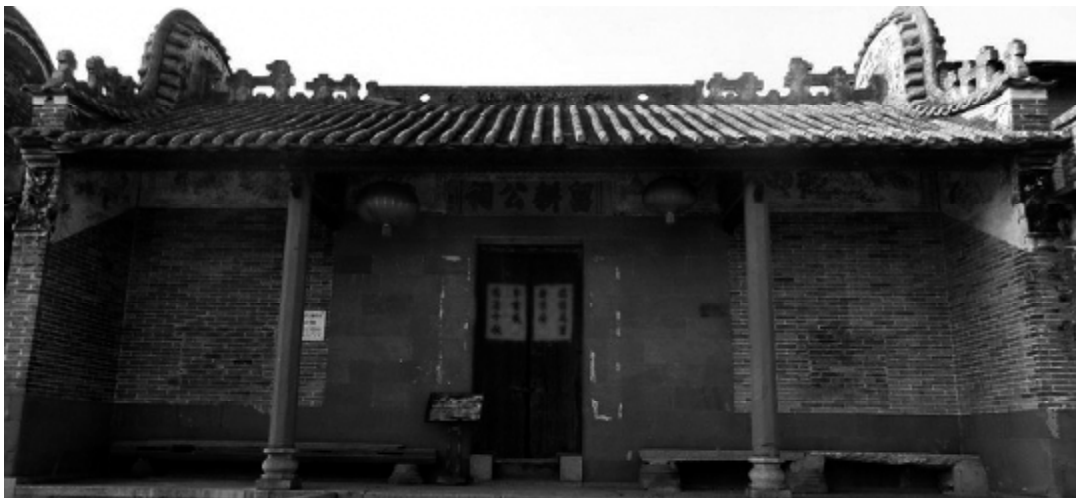
Figure 25. The pot-ear gable and Bogu ridge in Liugeng Ancestral Hall, built in 1799 and rebuilt in 1869 (Liu Shuting, 2008).
