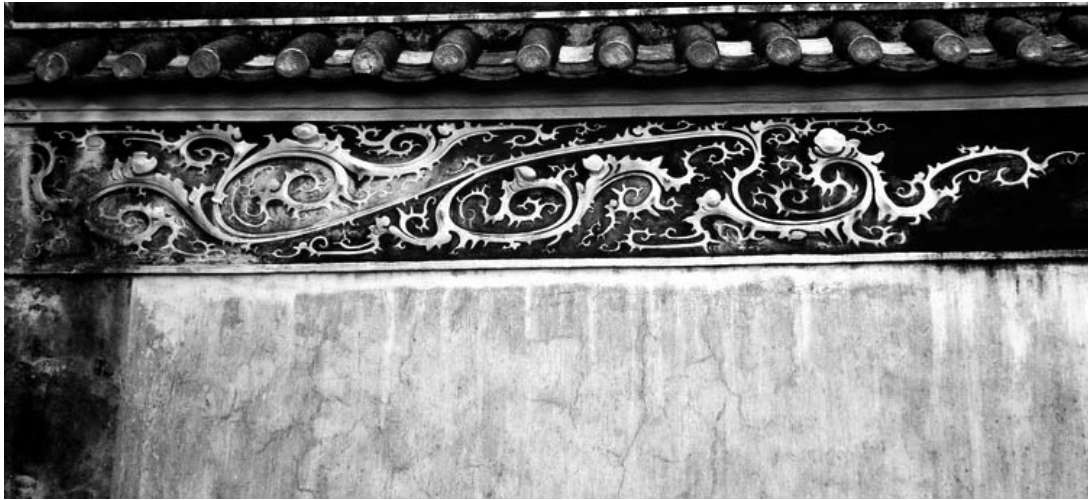
Figure 48. The bas-relief of scroll pattern on the on the Frieze of outer wall in Daling village in the city of Panyu.
