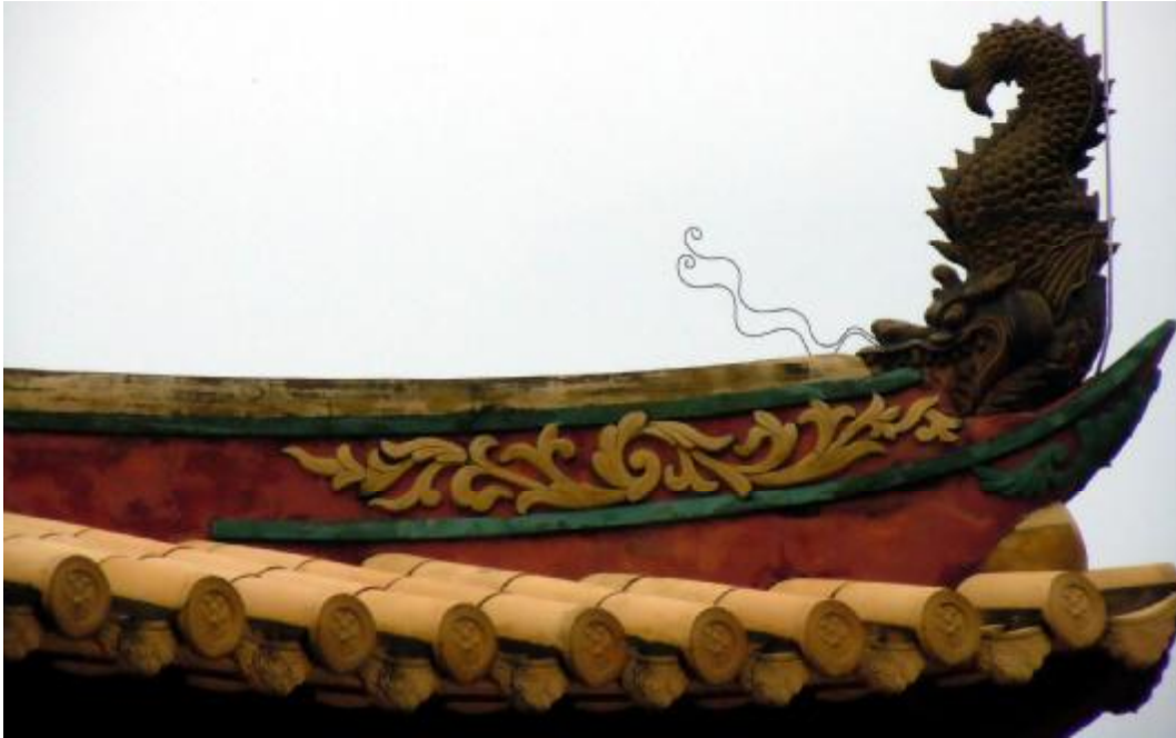
Figure 79. The decoration of Aoyu of the second eaves angle of hip roof in Mahavira Hall.
