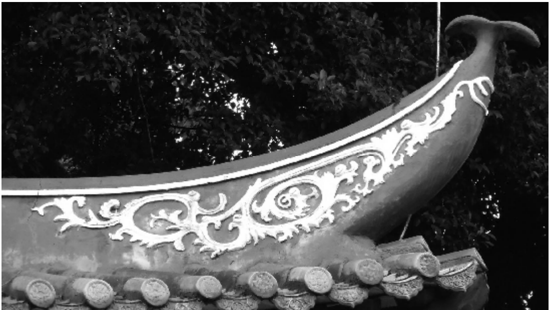
Figure 41. The fishtail-decoration on the hip of the roof of Jialan hall in the Guangxiao Temple (1611).
