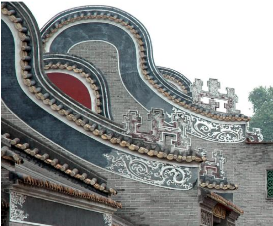
Figure 12. Low relief plaster with scroll design on gable wall in Fushan Ancestral Temple.
