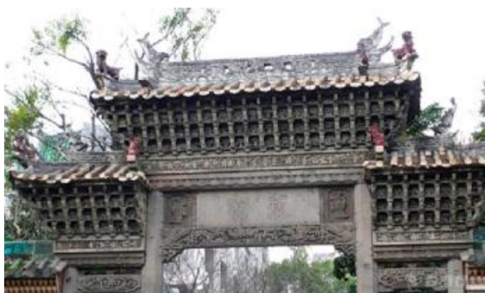
Figure 6. Low relief plasterwork in the main ridge of the roof on the Baochong Memorial Arch in Fushan Ancestral Temple in 1521.
