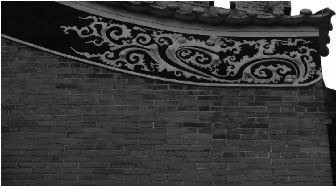
Figure 47. The bas-relief of scroll pattern on the gable wall of Qingzhen hall in Foshan Ancestral temple (1899).
