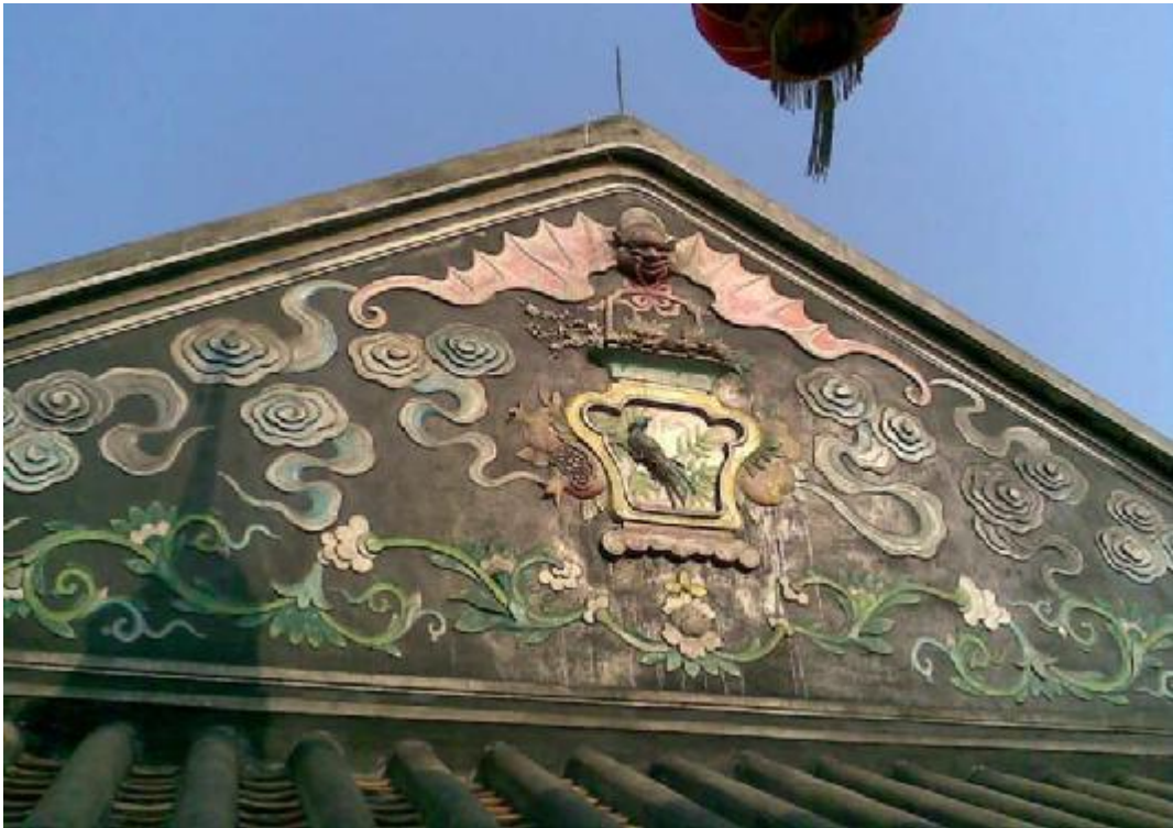
Figure 50. The plasterwork on the dutch gable of Shenliu hall in Yuyinshan garden In Panyu district (1871).
