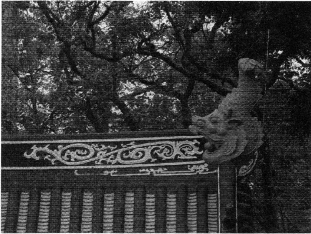
Figure 90. Aoyu plasterwork on the main ridge.
