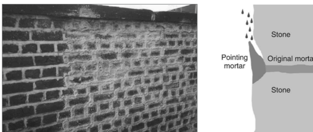
Fig 3.29 - Unaesthetic results of repointing (left) and example of wrong application of repointing [Bartuschka, 1995] (right).
