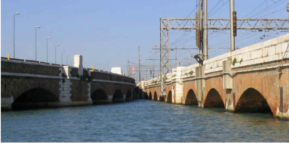
Fig. 4.6 - The only visible part of the old bridge, on the right, is the widening of the rail bridge close to Santa Lucia train station. The picture is taken when the road bridge, on the left, turns.
