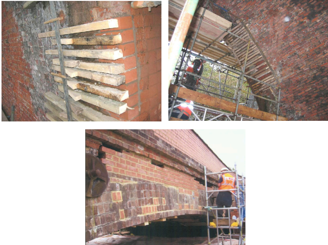
Fig 3.30 - Operation of patch repair of arch (above) and spandrel wall (below).
