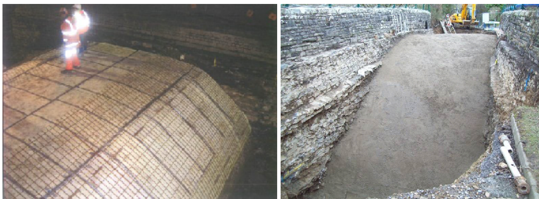
Fig 3.40 - Construction of concrete saddle.
