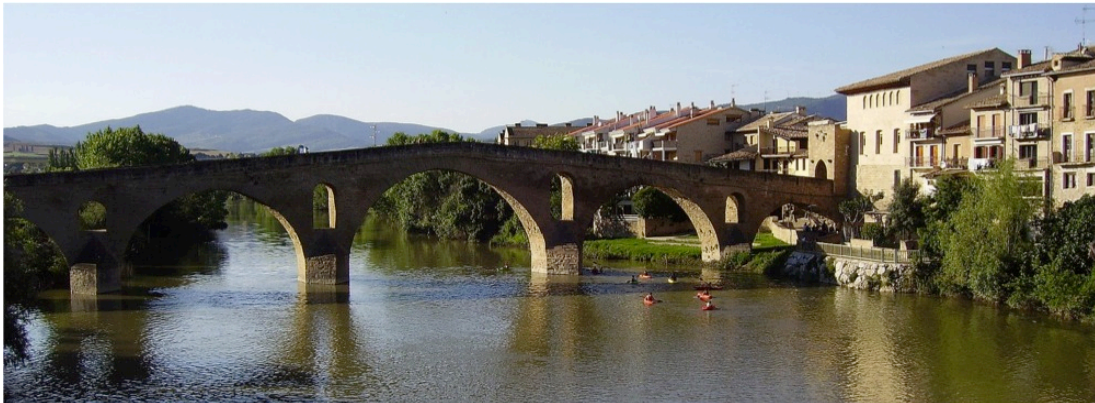
Fig 1.5 - Typical medieval bridge, Puente de la Regina, Navarra, Spain
