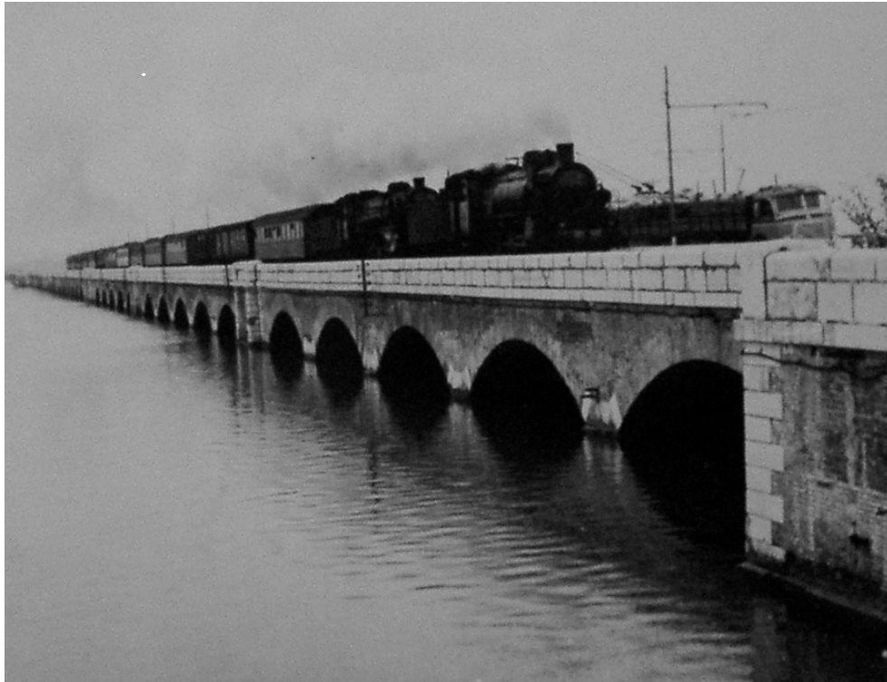
Fig. 4.3 The historical bridge in the XIX century.
