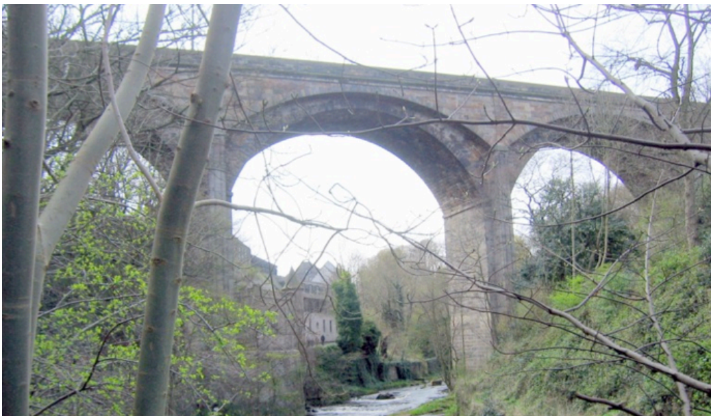
Fig. 1.17 - Dean Viaduct, Edinburg, Scotland.
