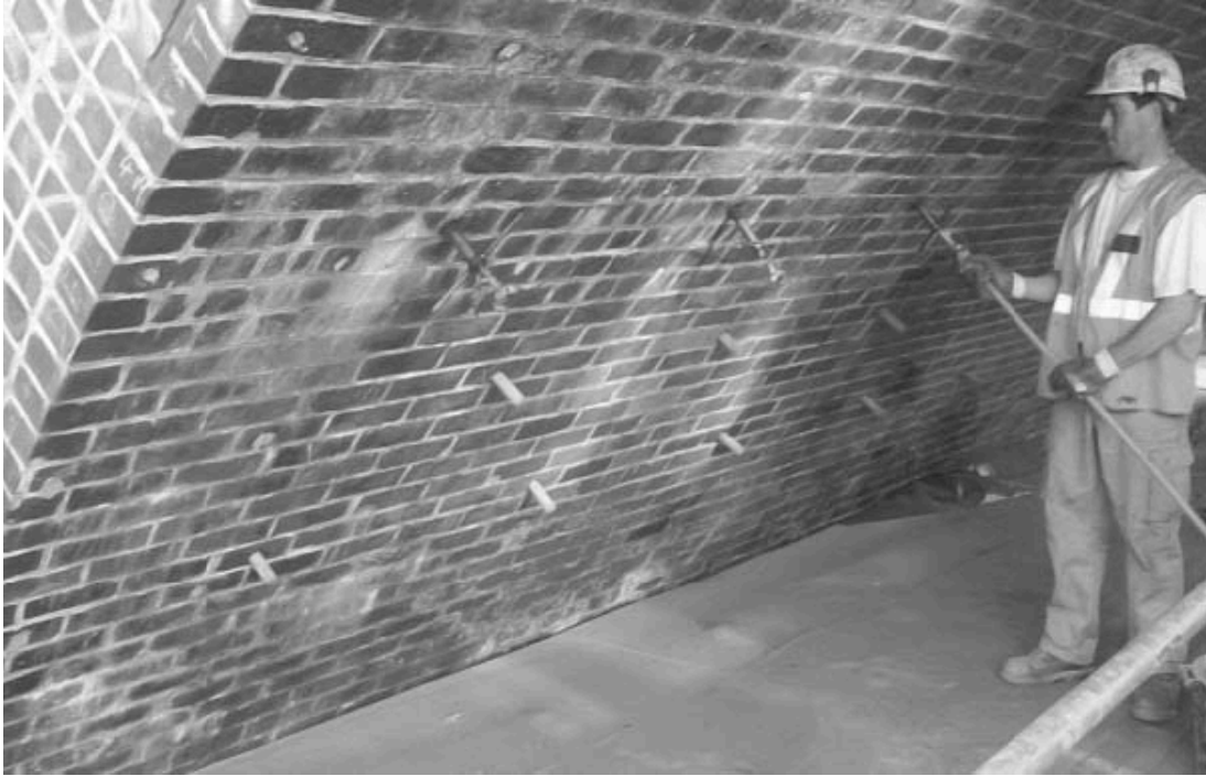
Fig 3.33 - Operation of arch grouting (taken from McKibbins et al., 2006).
