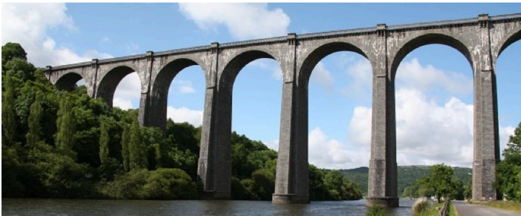
Fig 1.16 - Rail viaduct of Port Launay, France
