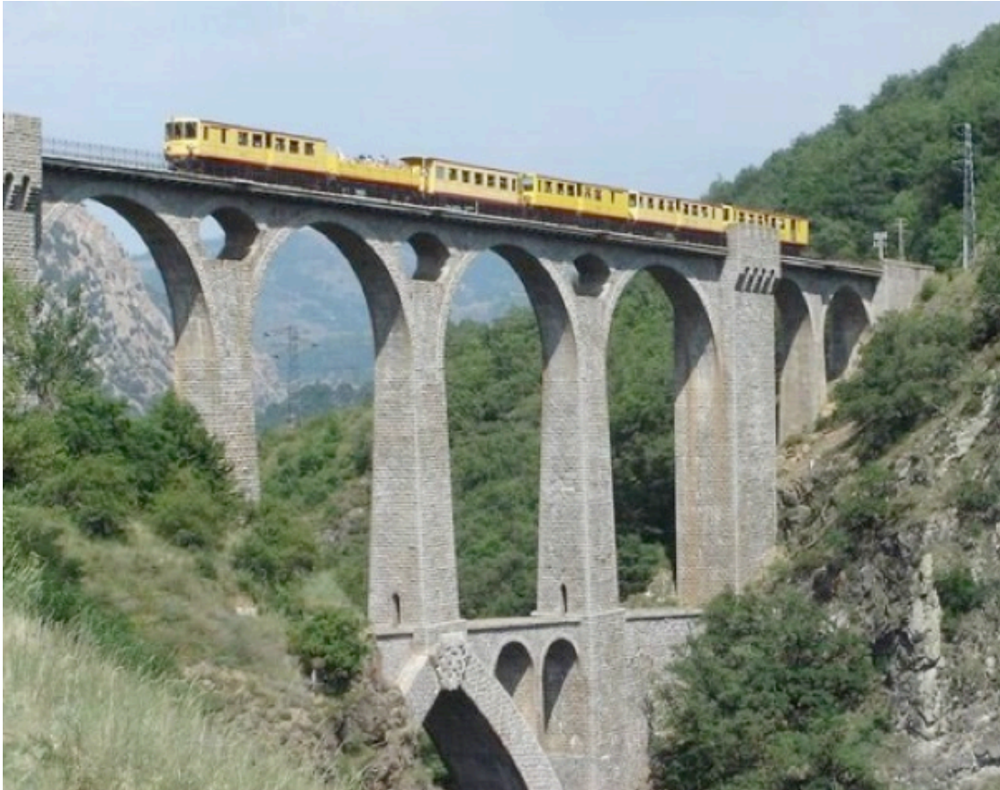
Fig 1.18 - Sejourne, Fontpederuse railway viaduct, France.
