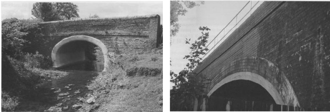
Fig 3.32 - Sprayed concrete lining, taken from [Page, 1996].
