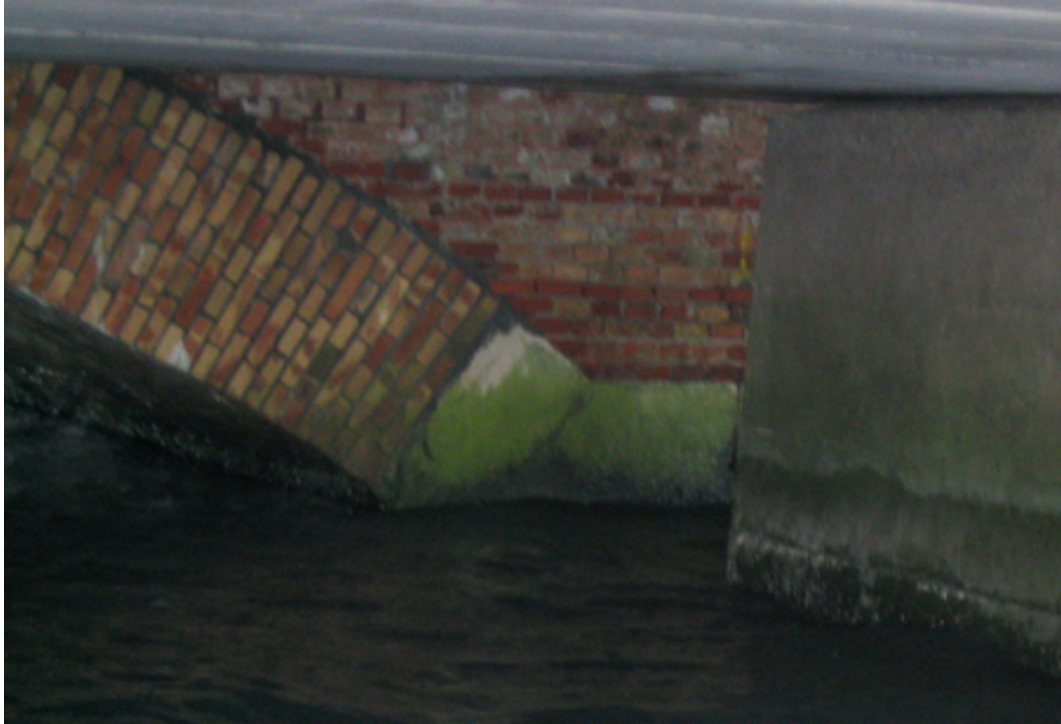
Fig. 4.48 - Particular of the 97 th arch: the texture of the original masonry
