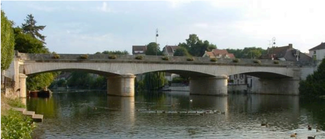
Fig 1.11 - Perronet, Pont de Neumurs, on the Loing River, France.
