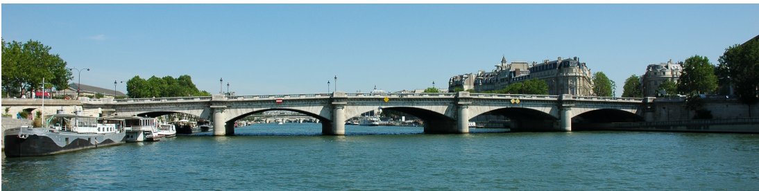
Fig 1.12 - Perronet, Ponte de la Concorde, Paris, France.
