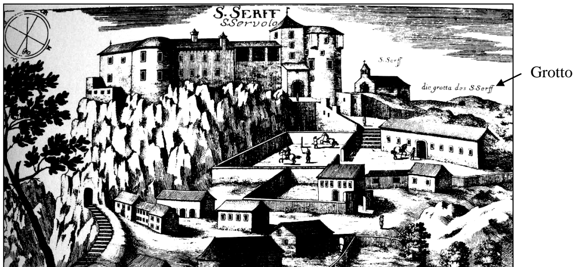
Figure 153 – Drawing from Valvasor (1689) which shows the Castle of Socerb and the Grotto of Saint Servolo to the right and back of the picture (Fister, Lah & Štupar-Šumi 1997, 238).
