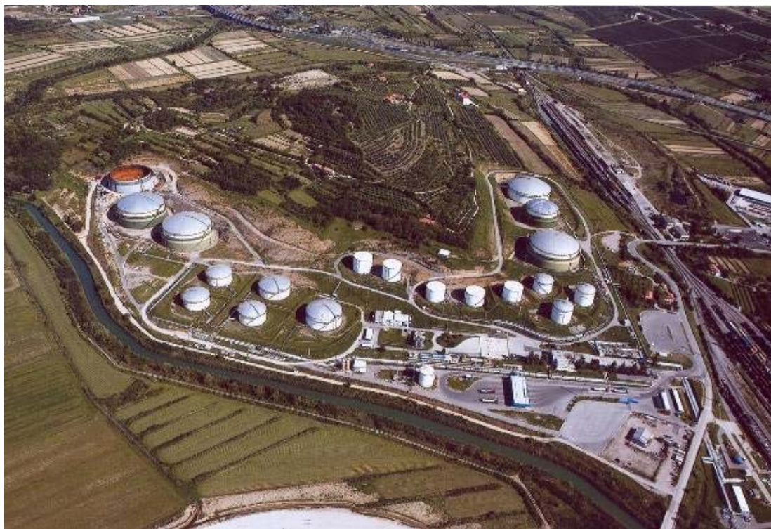
Figure 9: Panorama of Instalacija, storage and handling of petroleum products
