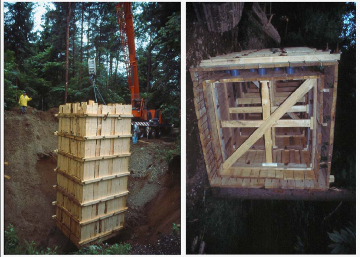
Figure 20: Lysimeter construction
