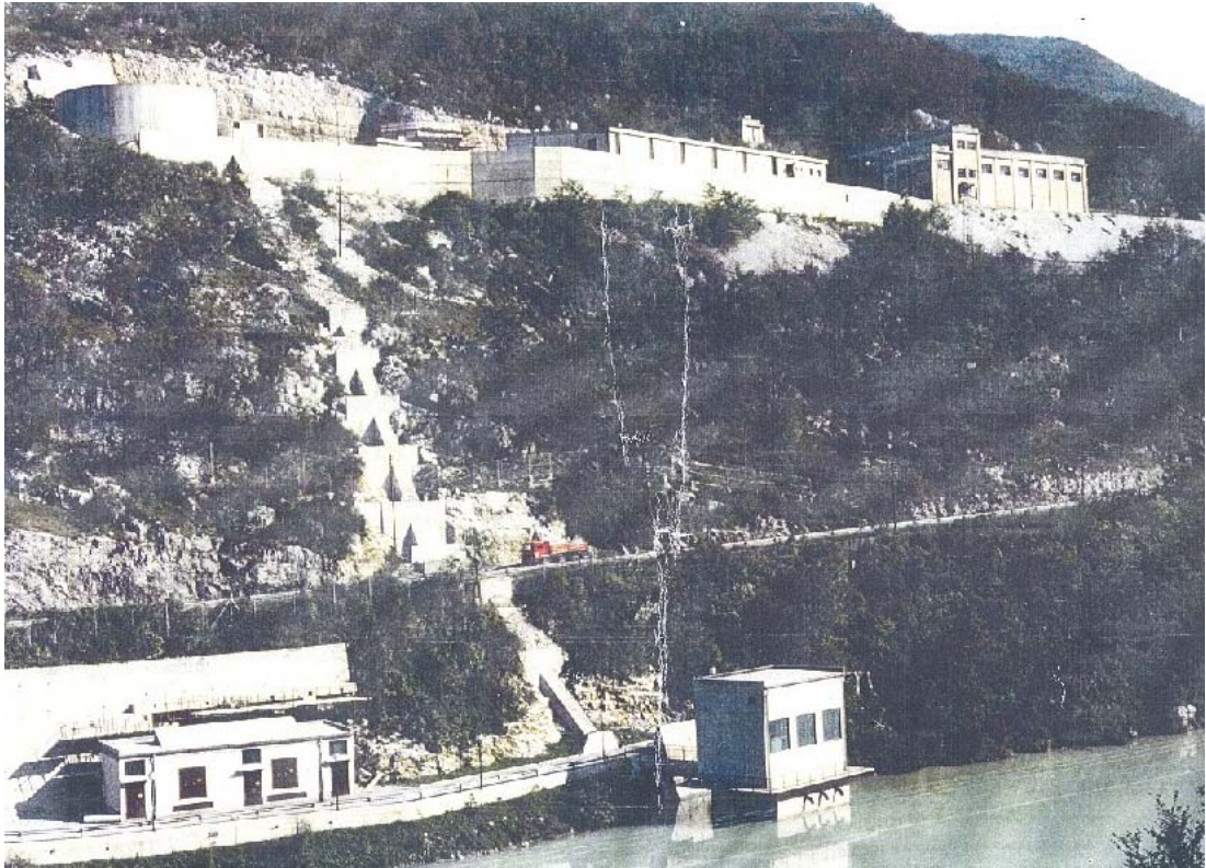
Figure 3: Mrzlek Waterworks pump station
