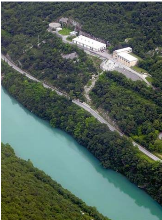
Figure 4: The old and the new Mrzlek Waterworks
