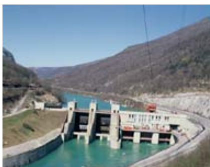
Figure 2: Solkan hydroelectric power plant
