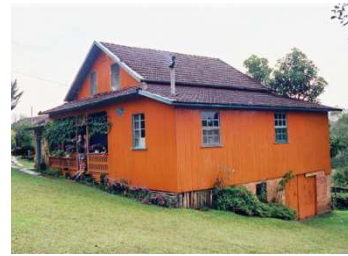
Picture 115 - House of Angelo Filipin in Crossroads São João. Source: PM-FR
