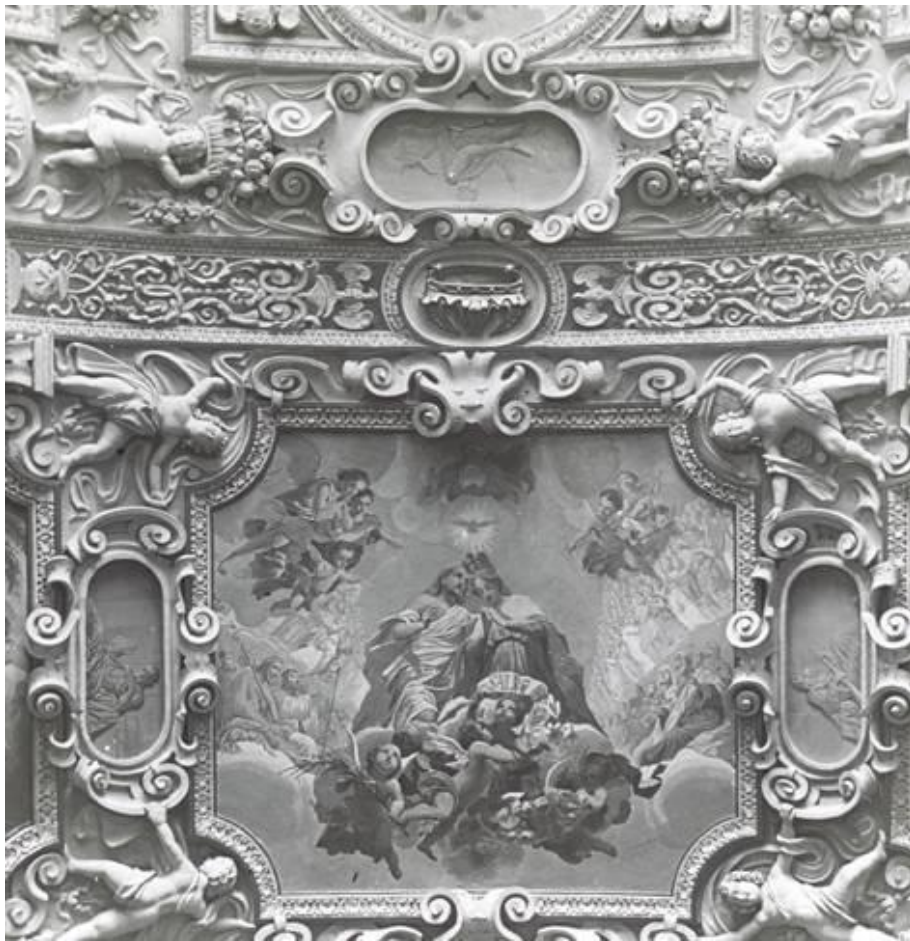
Fig. 4 Decoration of the vault of the central nave, before the I W.W.
