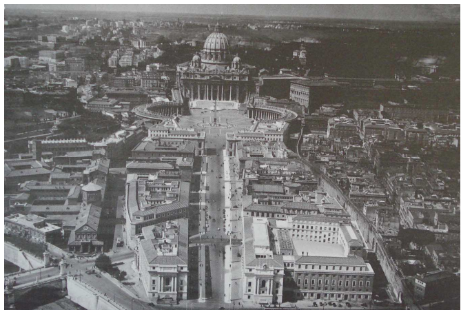
Image 5: View of the axial street opening up the St. Peter's Basilica to the River Tiber, in turn destroying the historic fabric in-between
