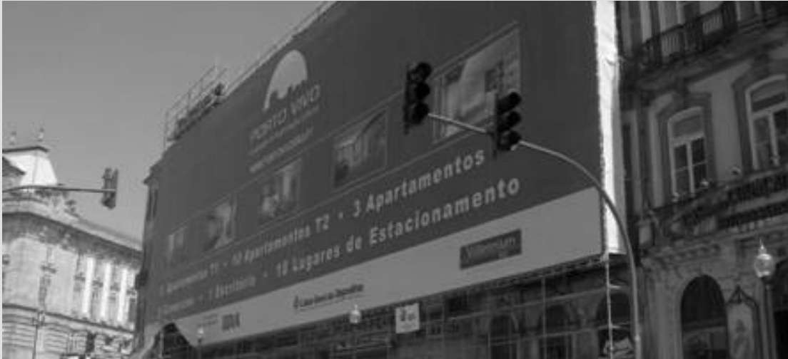
(IMAGE: PORTO VIVO SRU_REHABILITATION WORKS_SOURCE: INTERNET)
