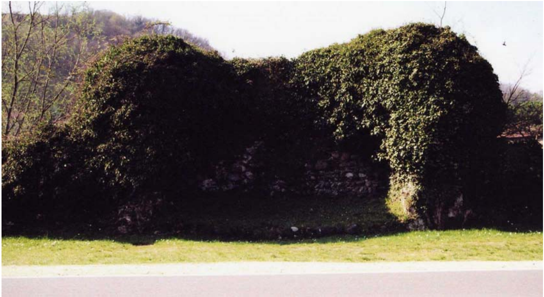
Illustration 11 - Thick vegetation that covers a large part of the Bridge
