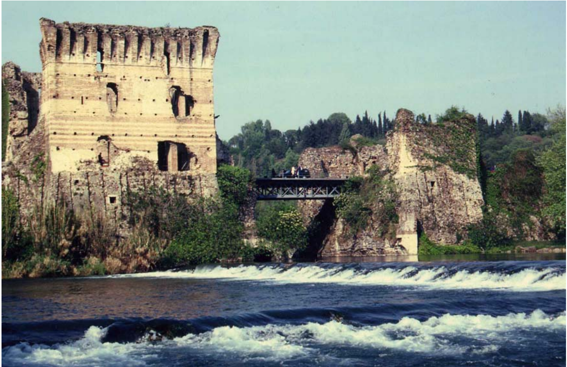
Illustration 1 – The bridge – dam of Valeggio sul Mincio (Verona)
