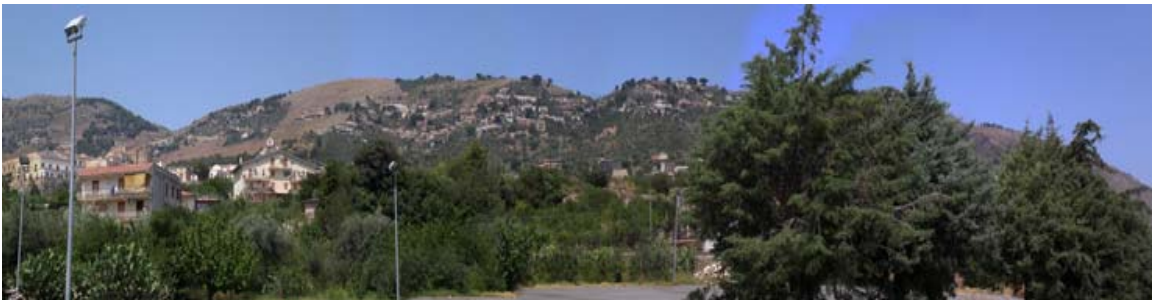
80 Housing above the city of Monreale.
