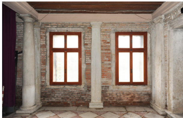
Image 75: Internal wall at ground floor
