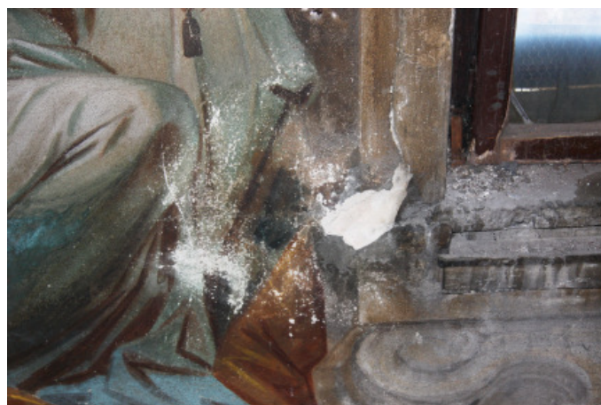
Image 98: Efflorescence, superficial erosion and lacuna
