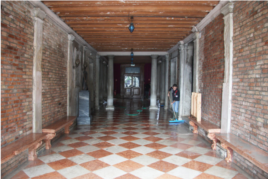
Image 68: Ordinary maintenance after flood tides
