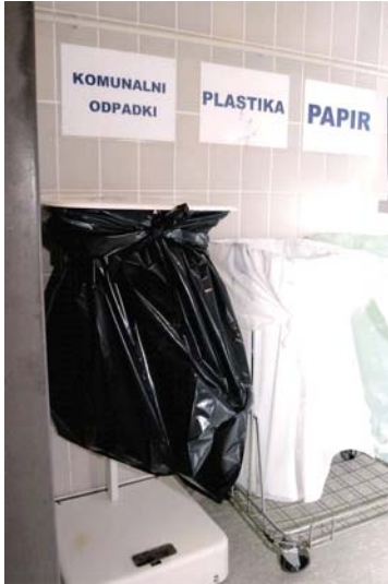
Figure 10: Unsanitary space in operation rooms (OP 3)
