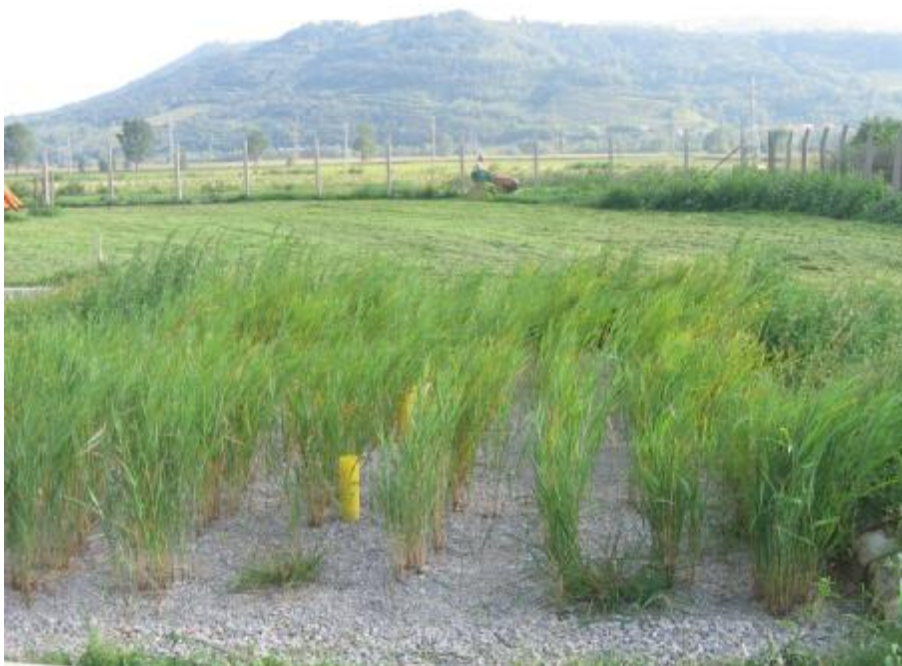
Figure 13: Wetland pilot plant in August with plants of Phragmites australis . Source-photo Lucija Kobal, 2004.
