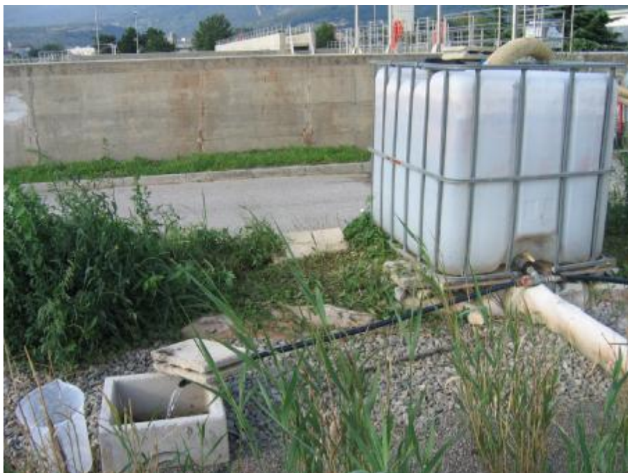
Figure 15: Regulation of inflow of waste water from the tank to basin A and B is regulated with inflow-valve. Source- photo Lucija Kobal, 2004.
