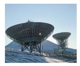
Fixed 42 m and steerable 32 m UHF parabolic antennas, Svalbard
